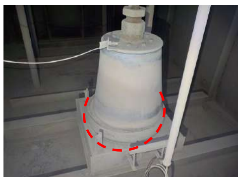
Fig.2 heater for supporting insulator
