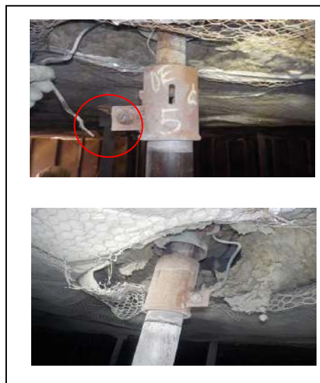
Fig.4 DE wire ground
